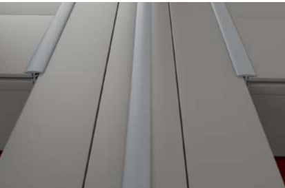
2 Multi-field system, connection point with rubber seal
